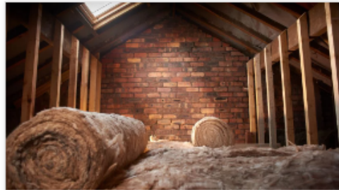
Weatherization and Insulation
