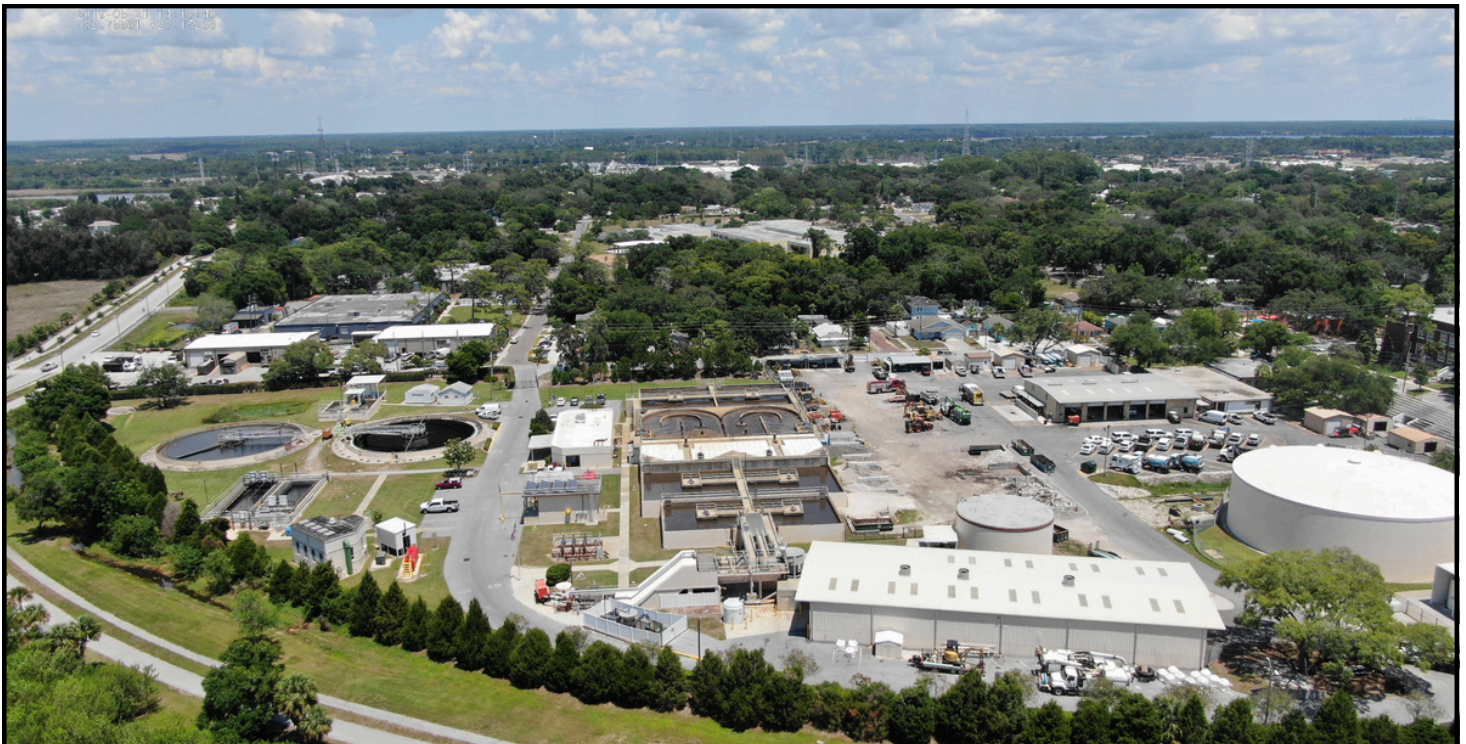
City of Tarpon Springs Advanced Wastewater Treatment Plant
