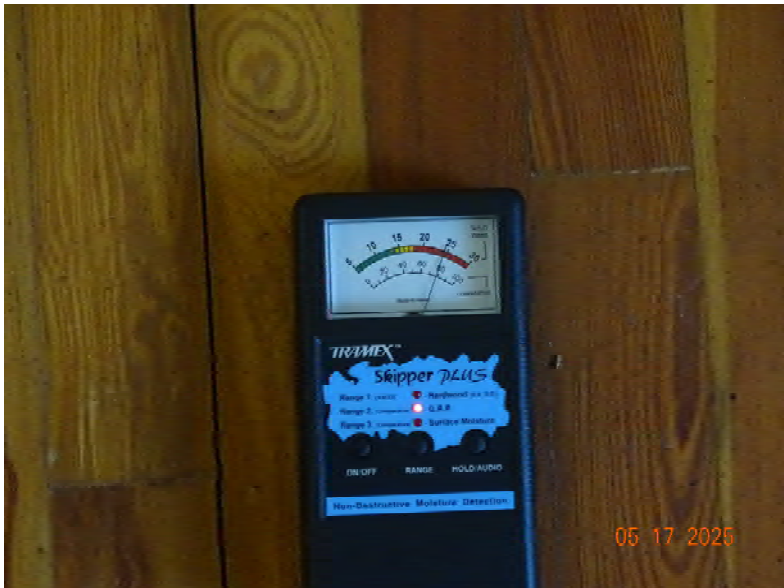
20 Moisture at floor
