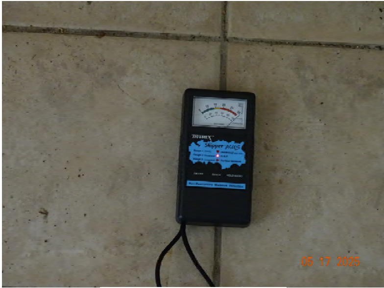
24 moisture at floor
