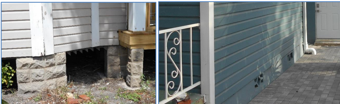
Figure 35. Support piers and continuous block walls are typical foundations used historically in the study area. The residence at 4 West Orange Street (left) used block piers, while the one at 18 North Ring Avenue (right) used a continuous block wall with decorative vents.
