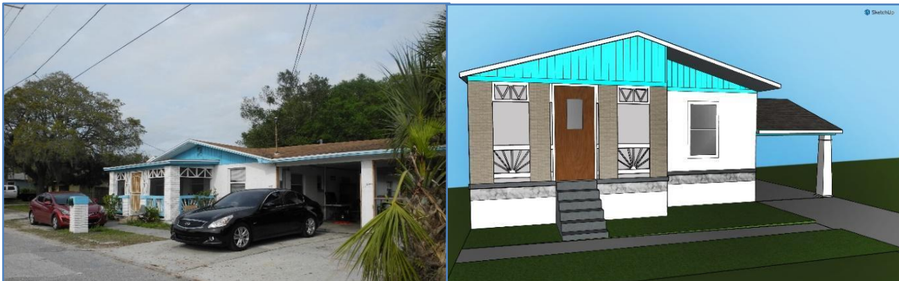
Figure 44. A slab on grade residence in the Union Academy neighborhood could potentially be elevated on foundation walls to the design flood elevation.
