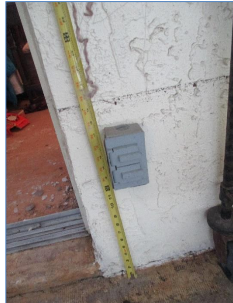
Figure 36. Twenty inches of floodwater covered electrical outlets at this mid-century slab on grade residence during a Category 1 hurricane (2016 photo).
