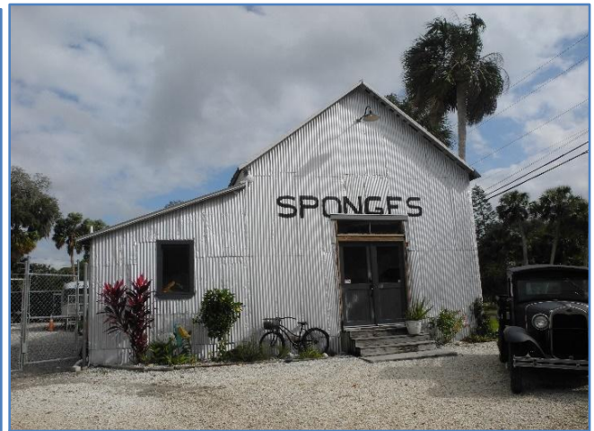
Figure 12. Meres Packing House, 2022 photo.
