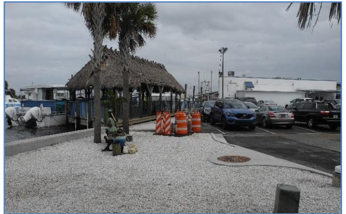
Figure 5. Sponge Docks drainage improvement project, 2022 photo.
