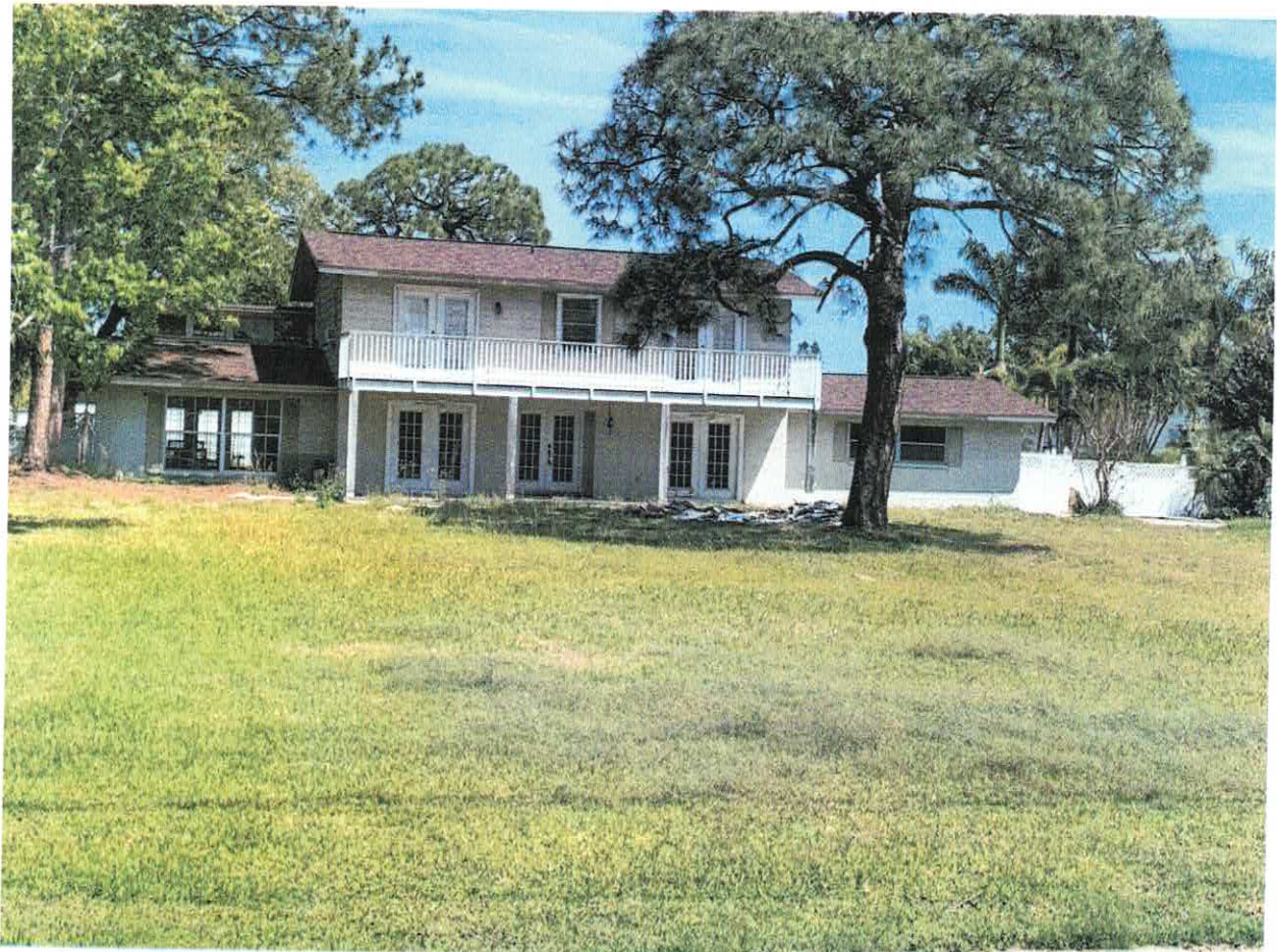
CASE # 25-80000476 SITE: 1019 S FLORIDA AVE TARPON SPRINGS, FL 34689 INITIAL INSPECTION BY CEO MROLLESTON: 4/1/2025
