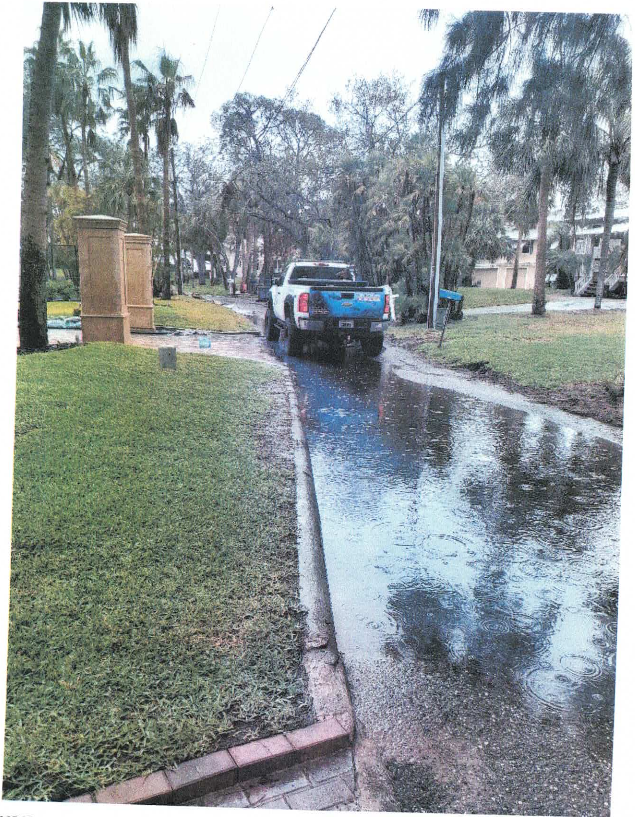
CASE 25-8000428 SITE: 1403 CIRCLE DR INITIAL INSPECTION 2/20/2025 STORMWATER - PAUL HOPKINS
