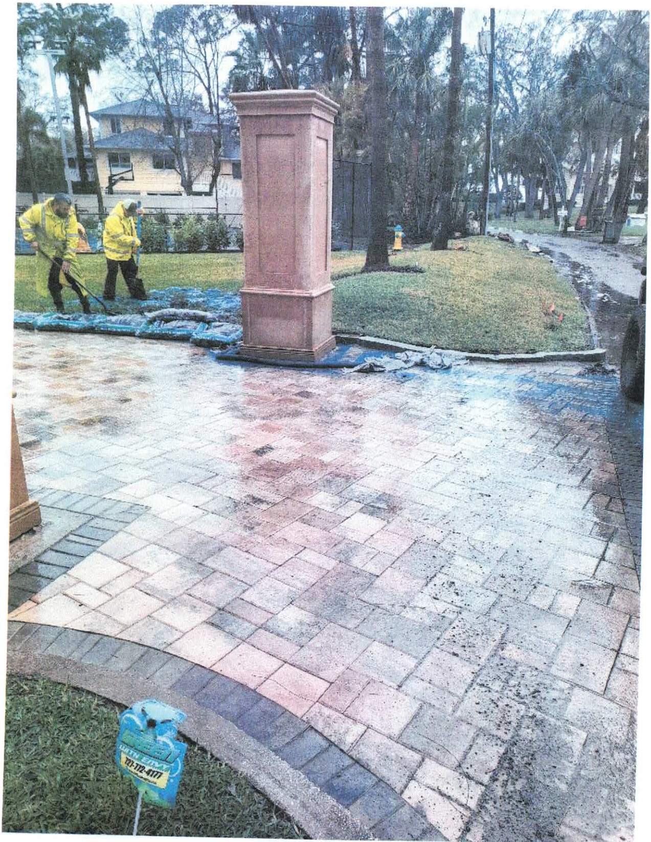
CASE 25-80000428 SITE: 1403 CIRCLE DR INITIAL INSPECTION 2/20/2025 STORMWATER - PAUL HOPKINS
