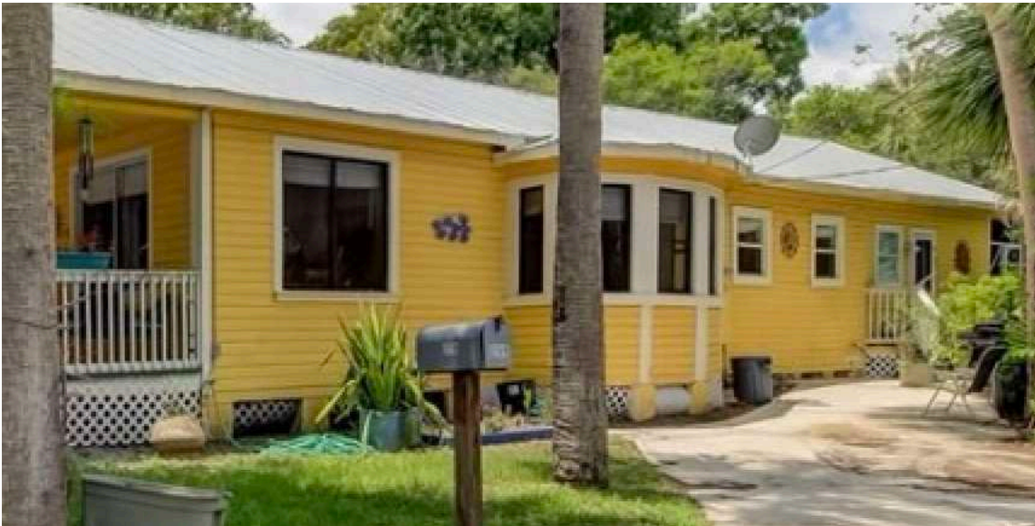
219 Grand Blvd/Gallagher Residence Existing unsympathetic windows
