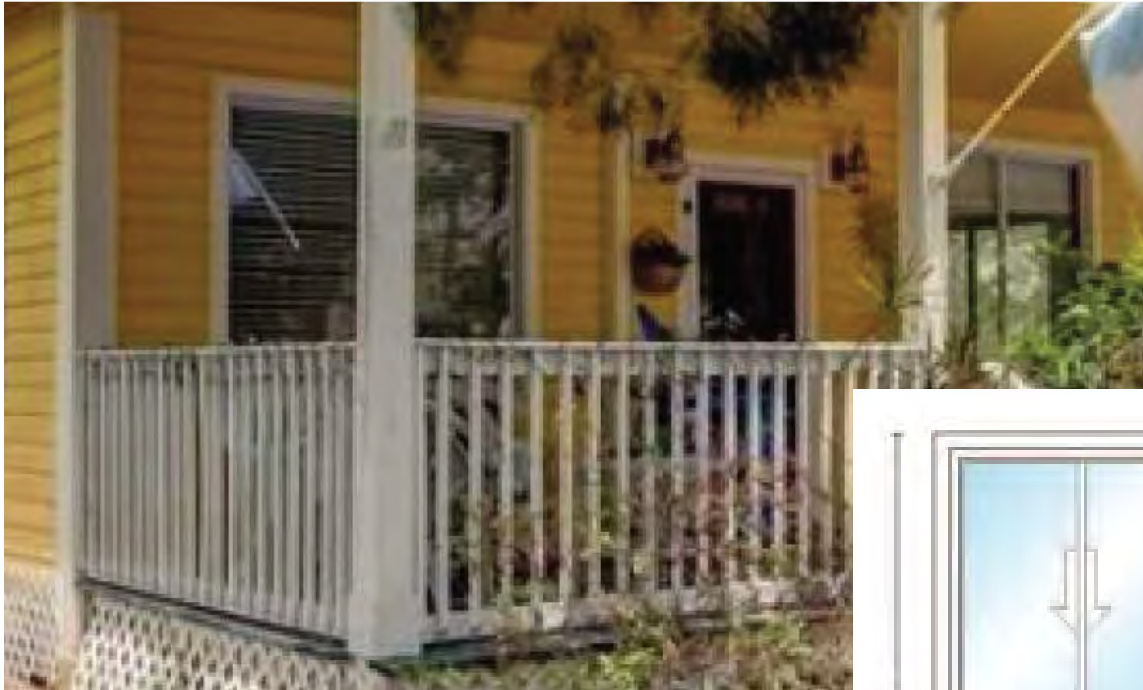
Façade Windows to be Replaced
