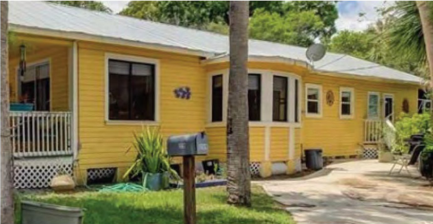
All Other Windows to be Replaced
