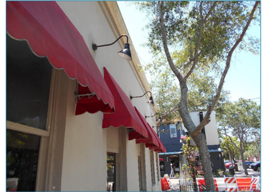
Figure 132: Awnings on 101 East Tarpon Avenue.
