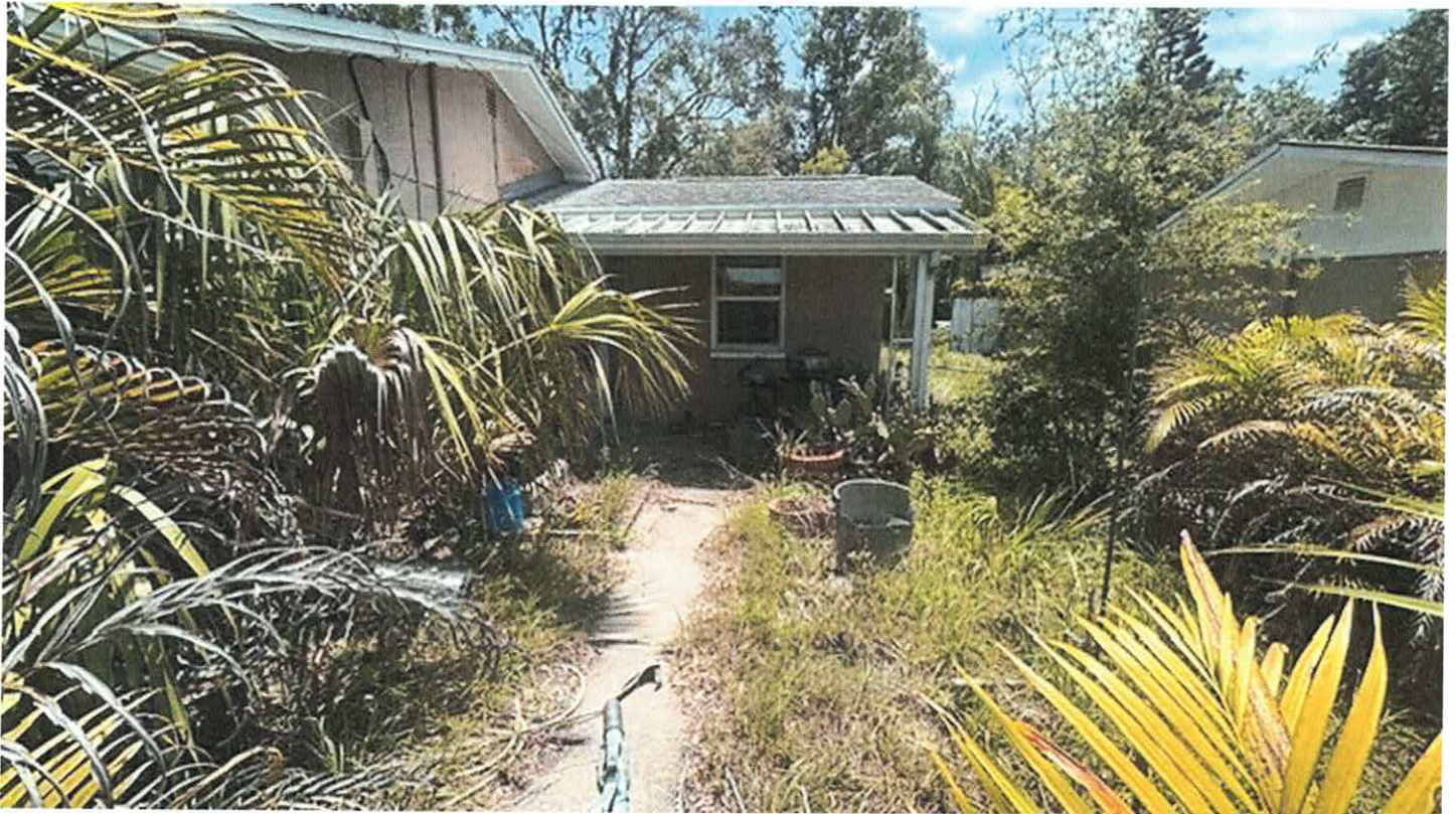
VIOLATION SITE: 307 SHADDOCK ST, TARPON SPRINGS, FL 34689 CODE CASE OFFICER: Michael Rolleston INITIAL INSPECTION 7/15/2026
