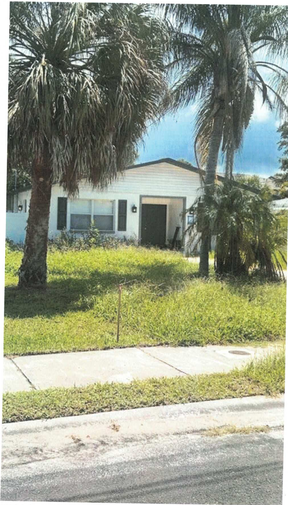
VIOLATION SITE: 715 VIRGINIA AVE, TARPON SPRINGS, FL 34689 Code Officer Anthony Boone Re-inspection 8/24/2026
