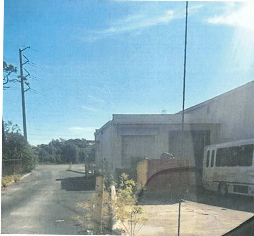
VIOLATION SITE: 1943 N PINELLAS AVE, TARPON SPRINGS, FL 34689 CODE CASE OFFICER: Anthony Boone INSPECTION 07/1/2026
