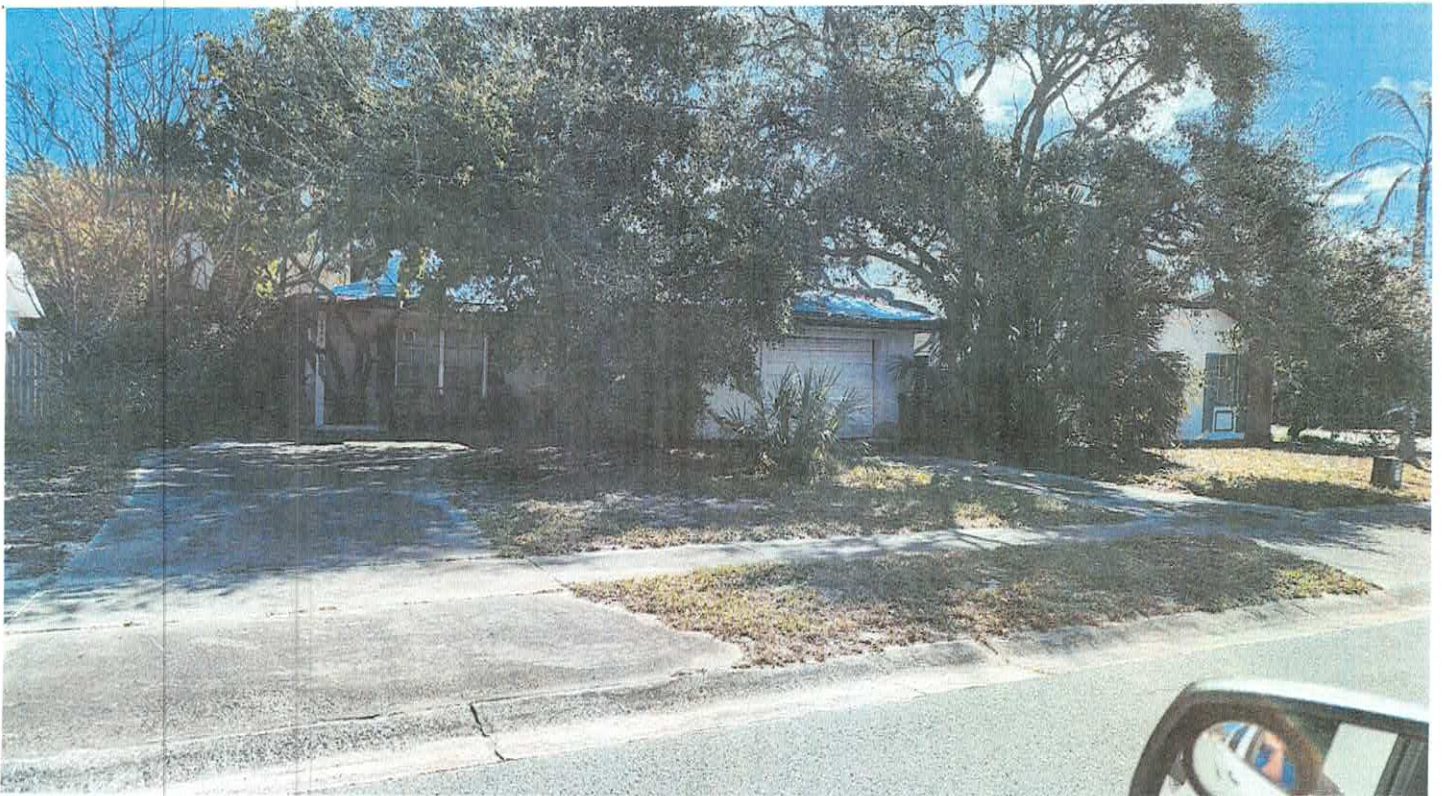
VIOLATION SITE: 1309 CROMWELL DR TARPON SPRINGS, FL 34689 INSPECTION 2/23/2026 BY CEO MICHAEL ROLLESTON
