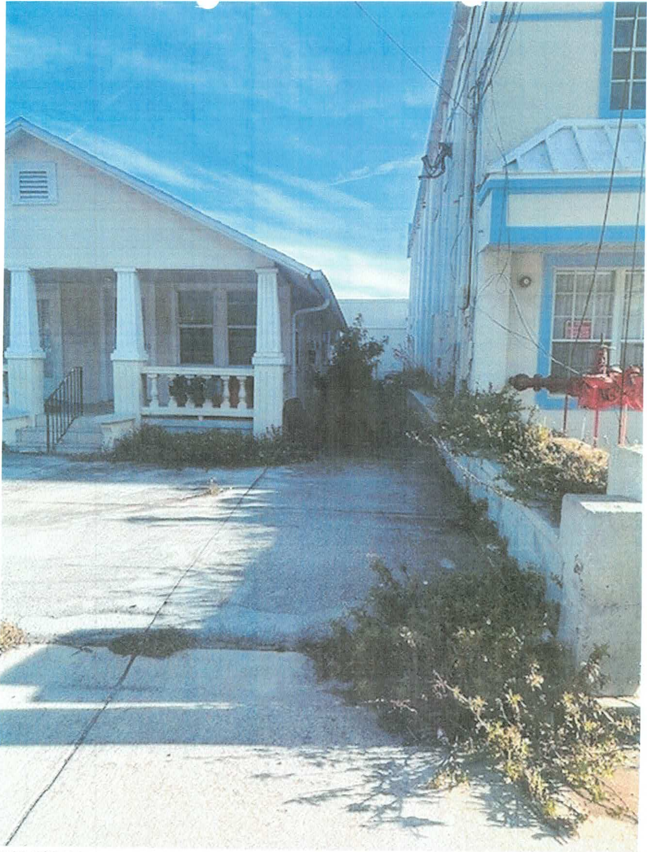
VIOLATION SITE: 120 ATHENS STREET, TARPON SPRINGS ,FL 34689 INITIAL INSPECTION 2/2/2026 BY CEO MICHAEL ROLLESTON
