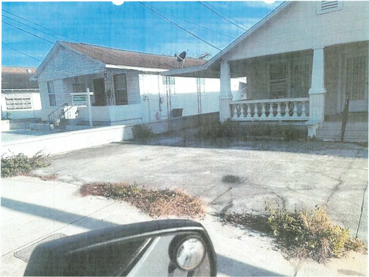
VIOLATION SITE: 120 ATHENS STREET, TARPON SPRINGS ,FL 34689 INITIAL INSPECTION 2/2/2026 BY CEO MICHAEL ROLLESTON
