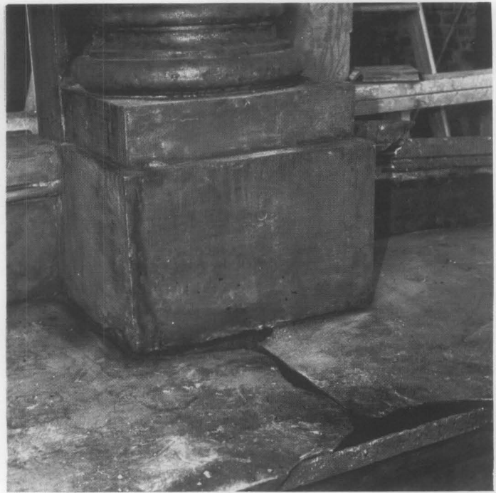
Fig. 12. Paint stripping exposed a large defect under a faulty patch at a joint of this wide cast-iron watertable. The damage can be repaired mechanically by splicing in a cast-iron replacement piece. Photo: Peter Jensen, Kapell and Kostow Architects.
