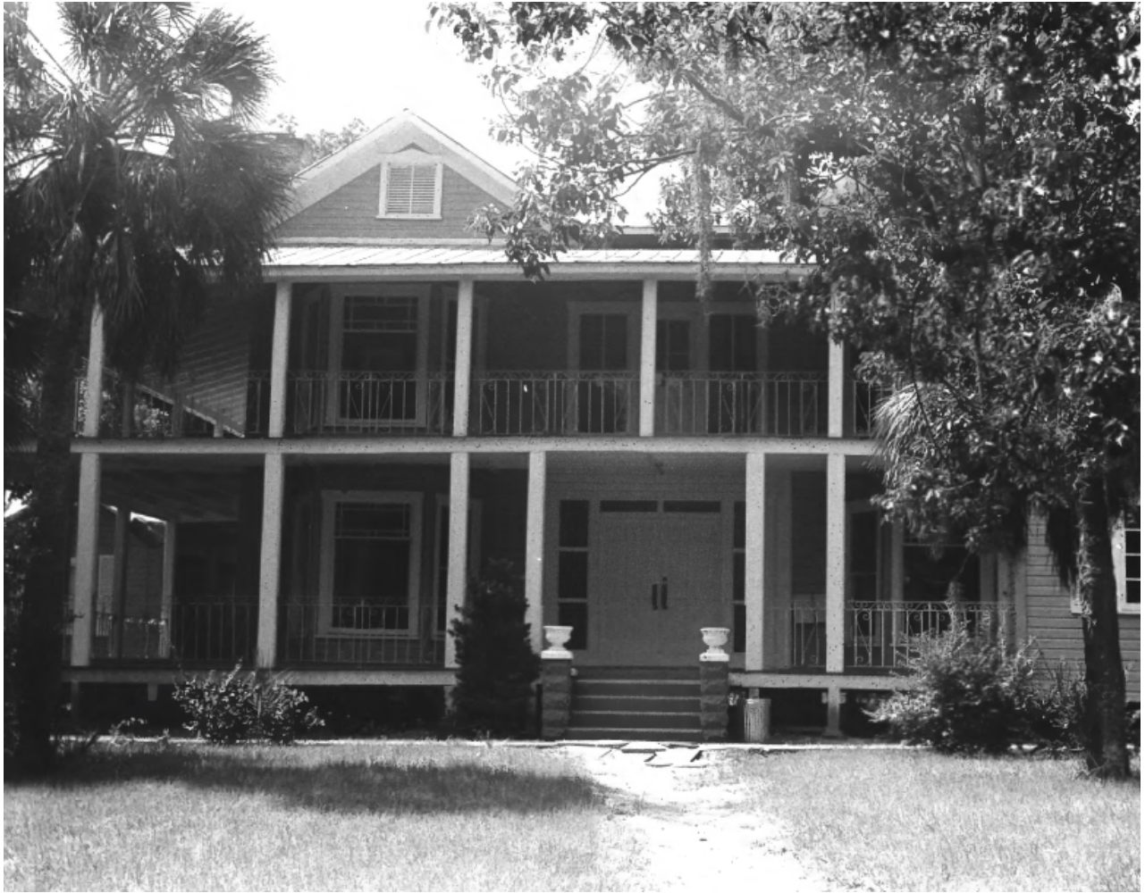
Figure 4. Safford House in 1973; note standing seam metal roofing on second-story porch (Safford House NRHP Nomination 1974).
