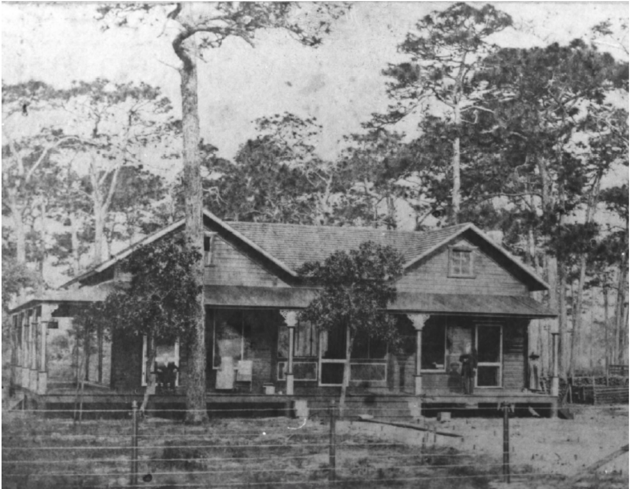
Figure 1. Safford House before 1887; note use of wood shingles on the primary roof (Safford House NRHP Nomination 1974).
