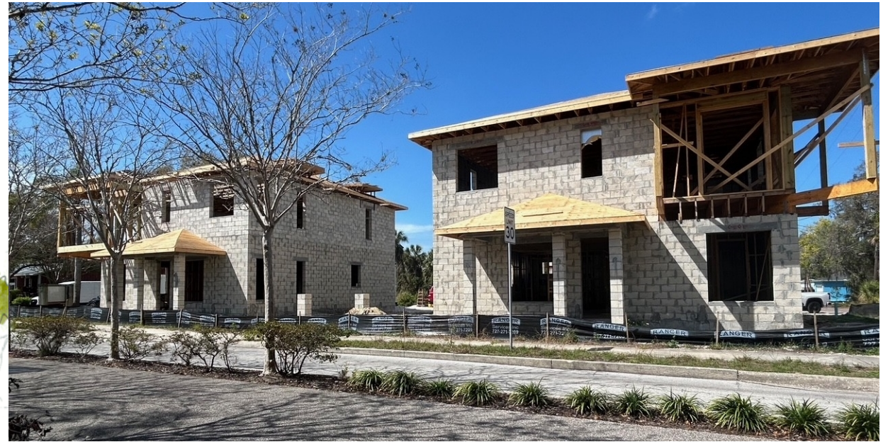
[Construction Progress March 2026]
