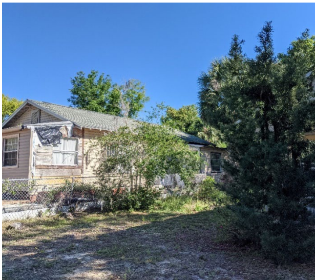
Figure 17 Historical home in disrepair.
