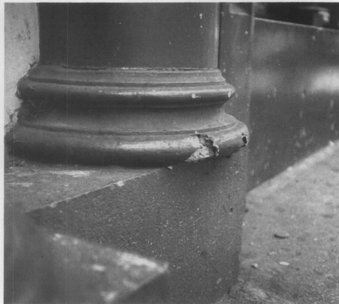
Fig. 20. The location of the feature must be taken into account if a substitute replacement material is being considered. This lightweight fiberglass column at street level sustained damage from impact within a few years of installation. The great strength of cast iron makes it ideal for storefronts and elements that must withstand heavy use. Photo: Building Conservation Associates.
