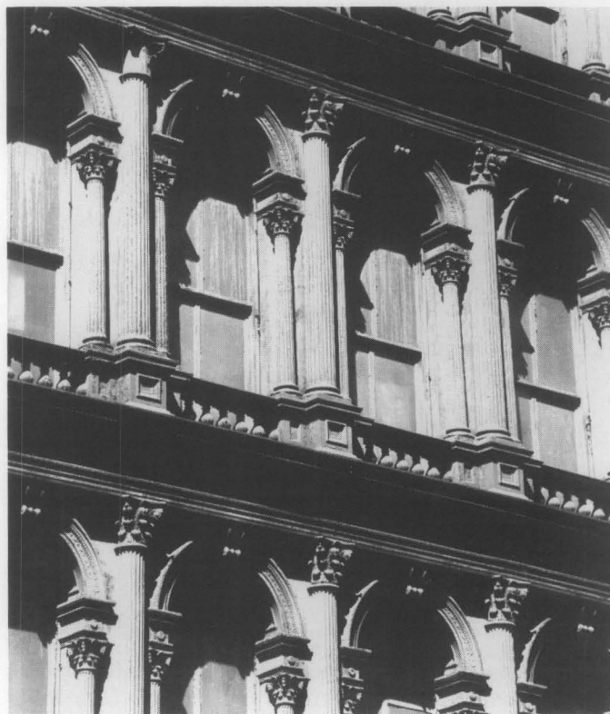
Fig. 1. The Haughwout Building in New York City is an excellent example of the quality and character of mass-produced cast-iron architecture. Once wood patterns were made, any number of elements could be cast, as was done with each of these repetitive bays. Photo: New York City Landmarks Preservation Commission.
