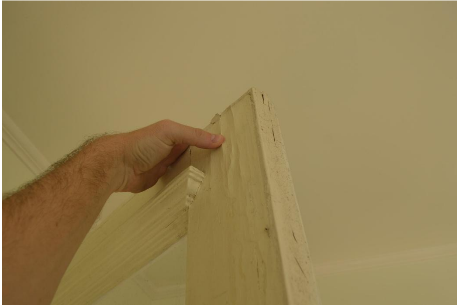
Photo 9: Damaged Exterior Wood Door (First Floor - South Elevation)
