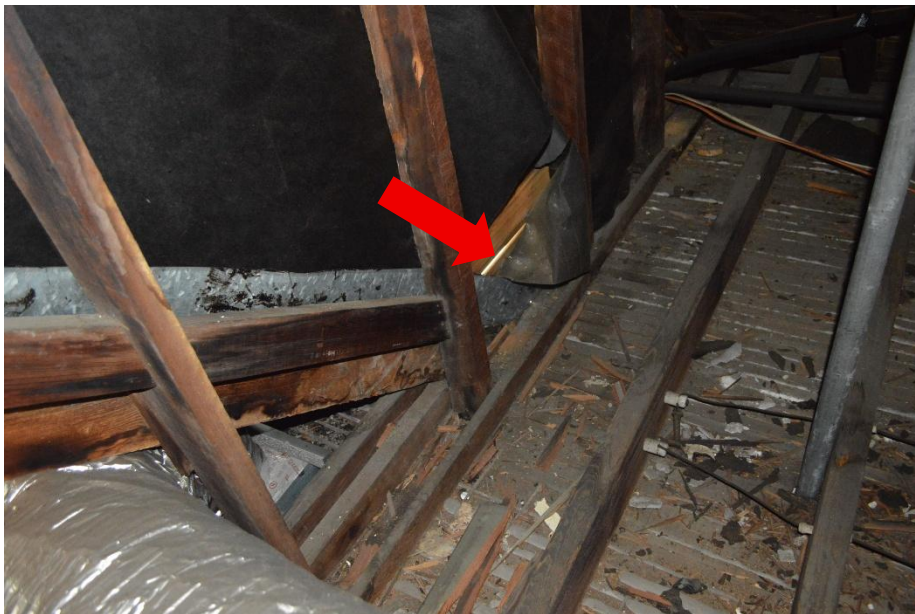
Photo 16: Opening to the Exterior in Attic (South Elevation)
