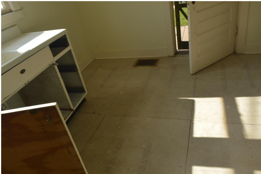
Photo 34: Unfinished Subfloor (Kitchen)
