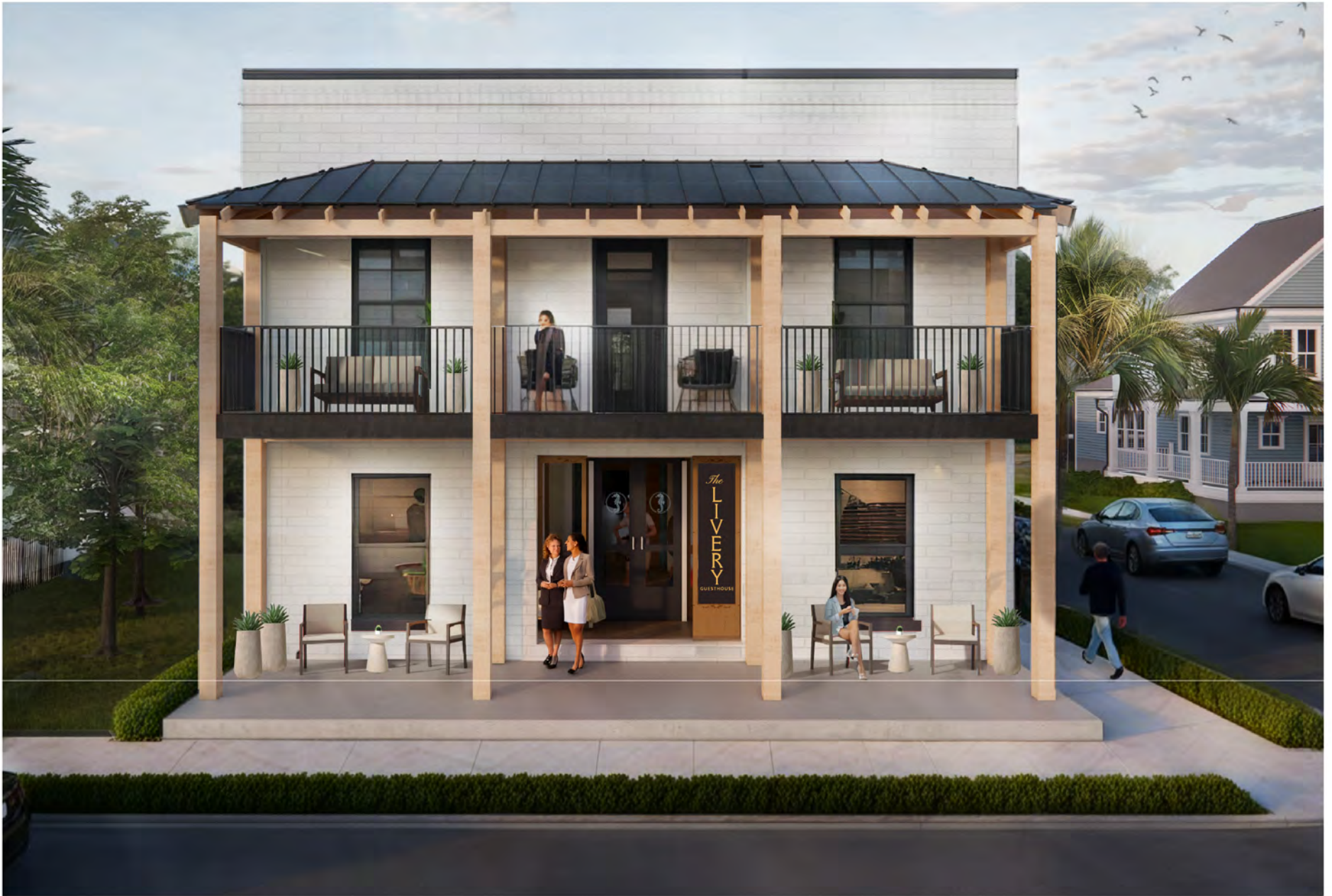
WEST SIDE - FRONT OF BUILDING
