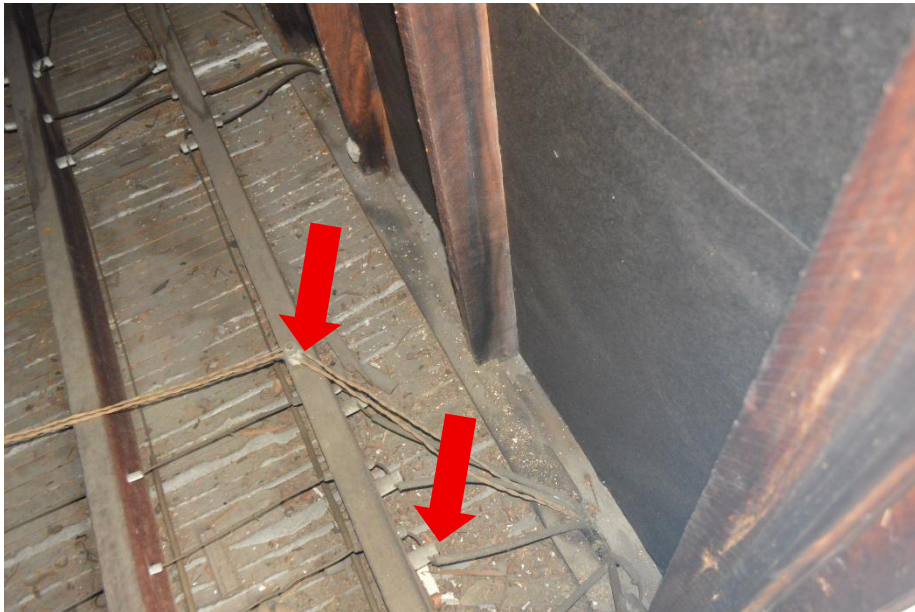
Photo 36: Knob and Tube Wiring (Attic)
