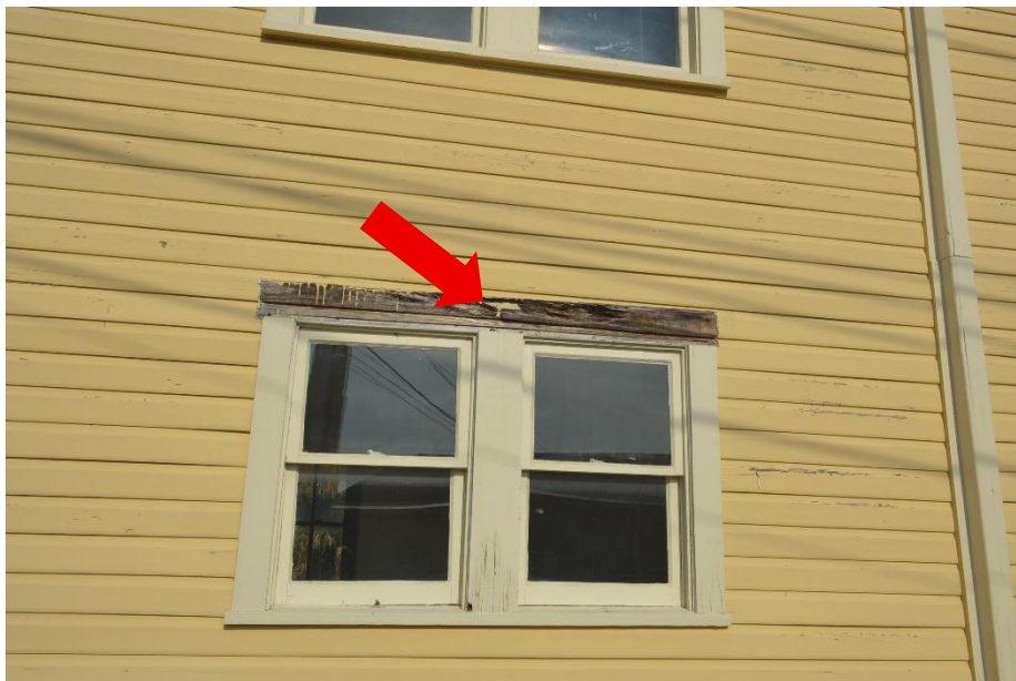
Photo 12: Exposed Exterior Outside of Kitchen (East Elevation)
