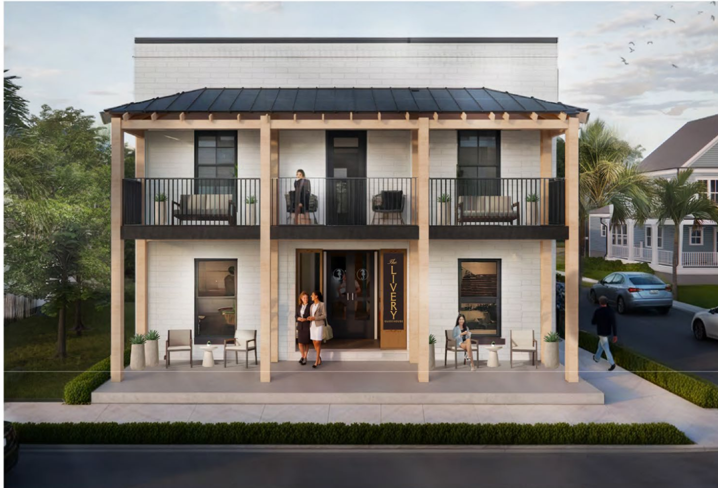
WEST SIDE - FRONT OF BUILDING
