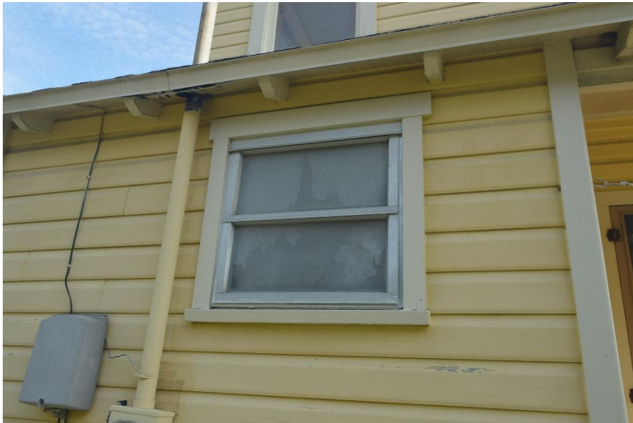
Photo 8: Aluminum Window (South Elevation)
