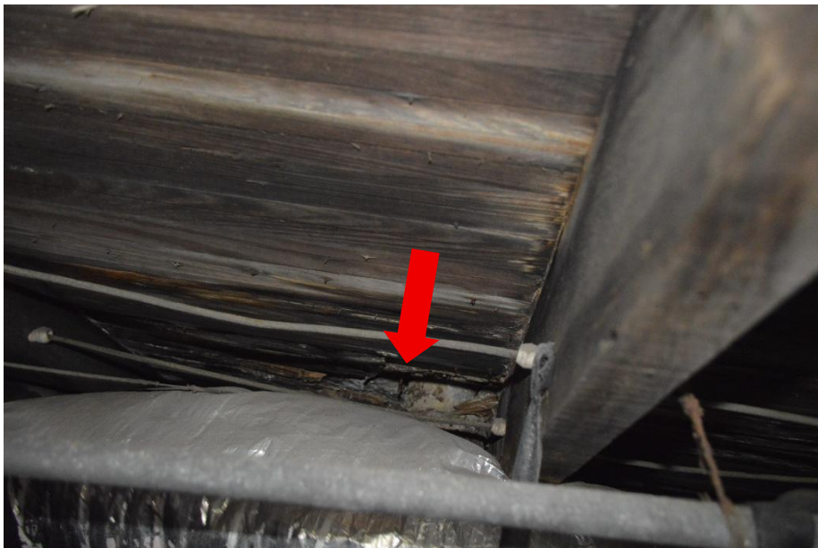
Photo 38: Rotted/Damaged Subfloor
