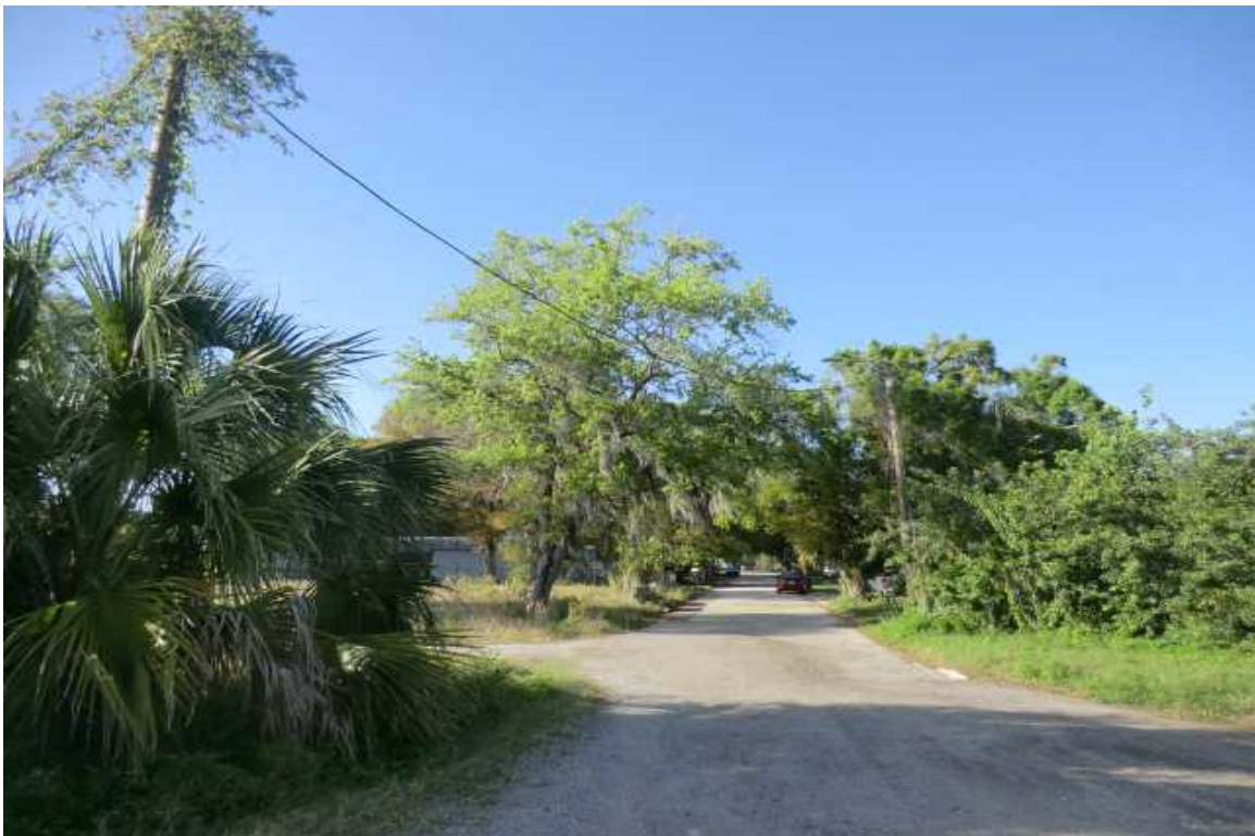
LINCOLN AVENUE - FACING NORTH
