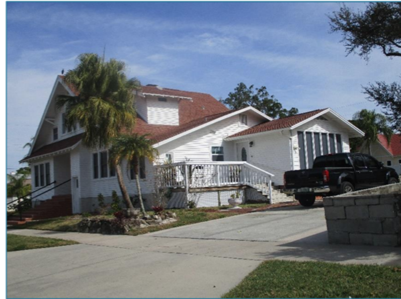
Figure 90: Multiple additions on the rear of 201 Bay Street are clearly subordinate to the original part of the building.
